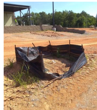
SILT FENCE AROUND
