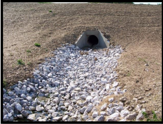
Rock used to slow water down at outfall
