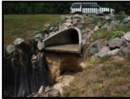
Severe Erosion from unmaintained outfall
