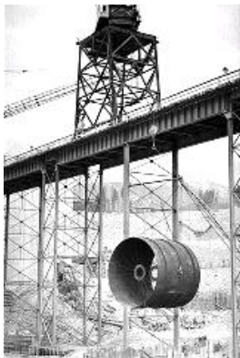
THE PENSTOCK: The pipe that collects water from a lake, reservoir or river and funnels it to the turbine. Penstocks are typically located deep in a lake and can have a large diameter. The penstocks at J. Strom Thurmond Power Plant are large enough to drive a school bus through and collects water from approximately 90 feet below the surface of the lake. This photo was taken during dam construction in the 1940's.
