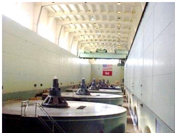
THE POWERHOUSE: The turbine, generator, and transformer are located in the powerhouse.
